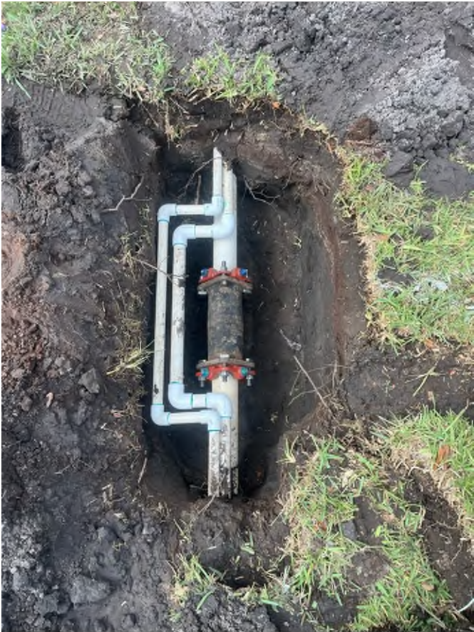
Mainline repair with 3" mechanical joint
