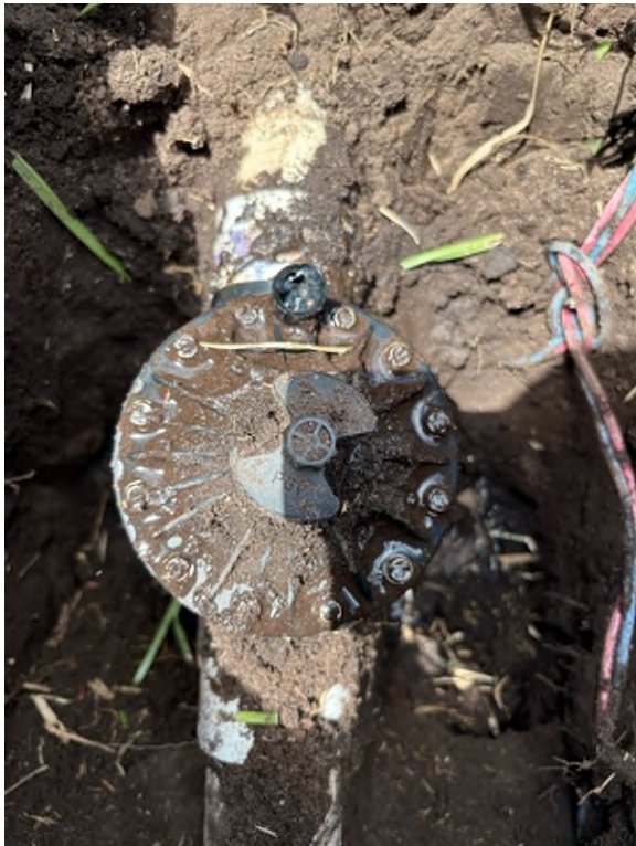
Replaced valve B56 with broken solenoid
