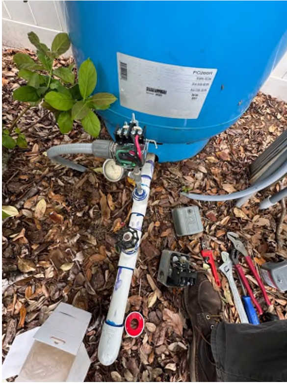
Replaced broken pressure switch
