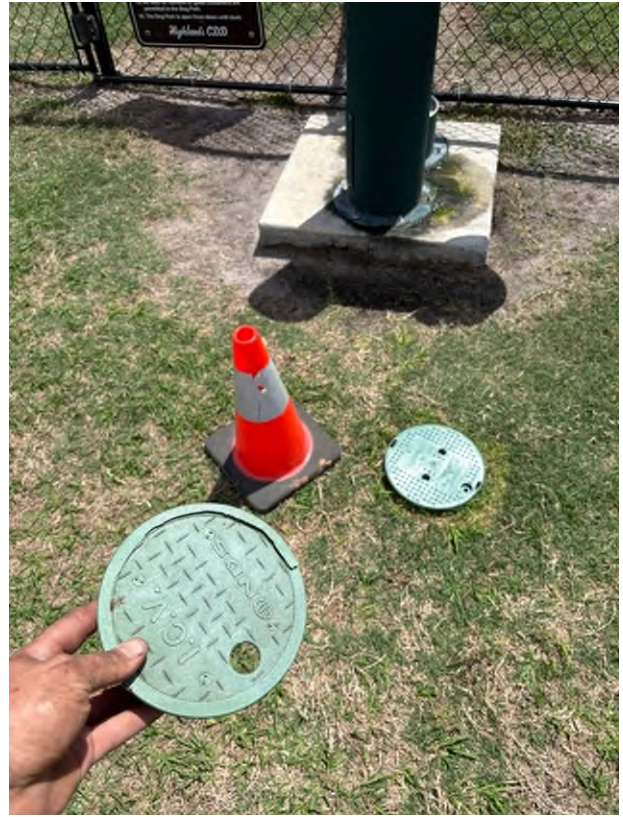
Replaced missing valve box lid
