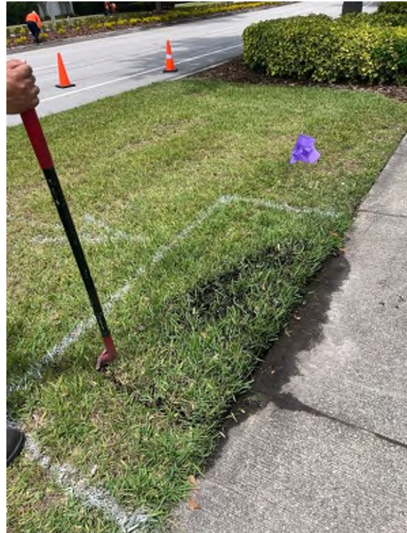
Mainline repair between Balm and Mystic Topaz
